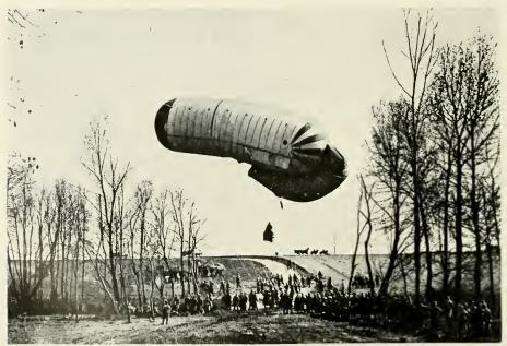
French observation balloon about to arise. The observer is in the "nacelle," or basket, suspended underneath and communicates with the ground by telephone. The large semicircular curved bag at the rear is open at the front to allow the wind to fill it and thus hold the balloon's head to the wind. A gasolene windlass on a truck hauls the balloon back to the ground when desired.
