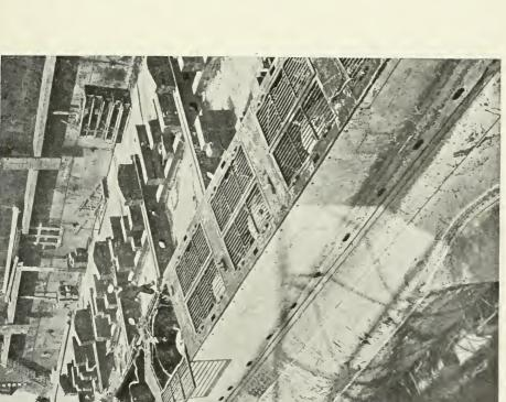
Mine-laying German submarine captured by the British. The mines with their anchors are in the grating-covered compariments. Their release is controlled from the coming tower.
