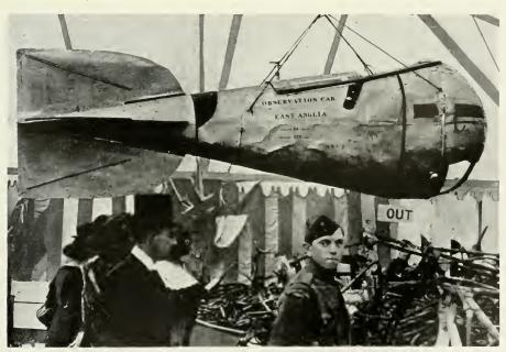
Zeppelin observation car. From a Zeppelin brought down in East Anglia: it is fourteen feet long, built of aluminium and weighs one hundred and twenty-two pounds. It was suspended by a wire cable 5,000 feet in length, through which ran a telephone wire. Observation windows are at the front and wertical and horizontal stabilizers at the stern.
