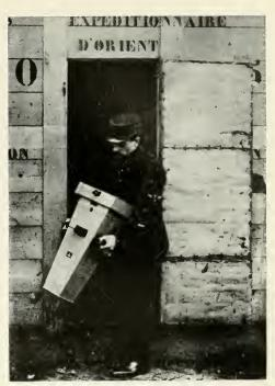
Apparatus used by the French for taking photographs from aëroplanes.
